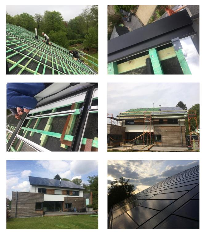
Figure 3.2: Installation and commissioning of Demo-system 1, Single House in Belgium
