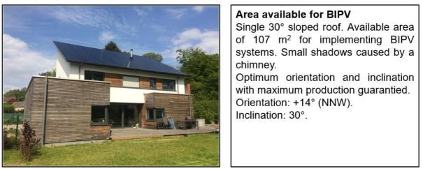
Figure 3.1: FD2: roof tiles system integrated at a single-family house in Belgium (resp: FormatD2)
