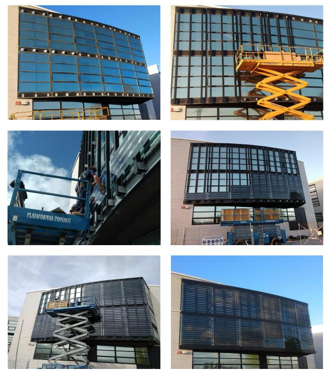
Figure 8.2: Installation and commissioning of Demo-system 6, Office Building in Spain
