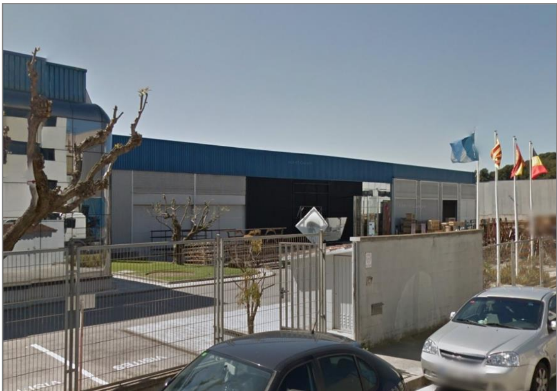
Figure 6.1: Industrial and office building complex in Spain, provided by CRICURSA.
