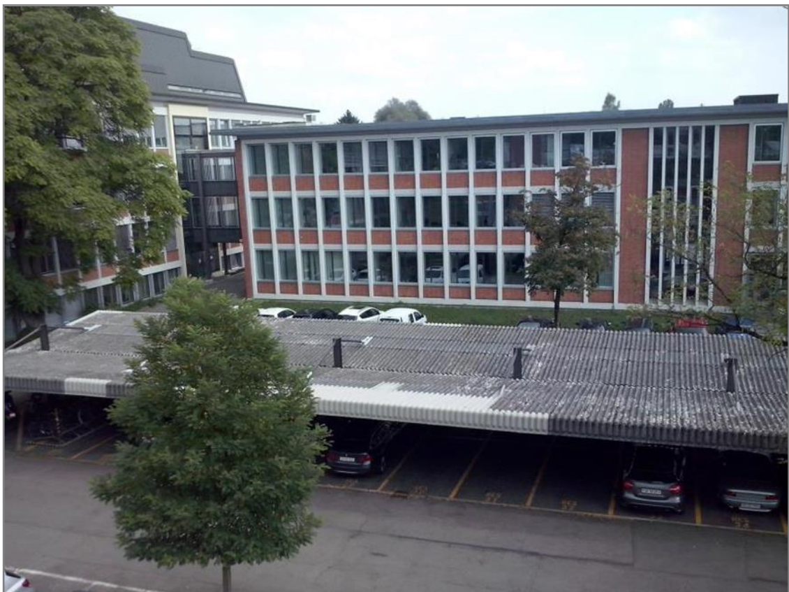
Figure 5.1: Public carport in Switzerland, provided by FLISOM.
