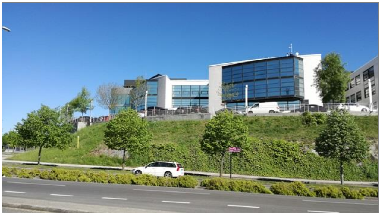
Figure 8.1: TECNALIA offices and labs in San Sebastian.
