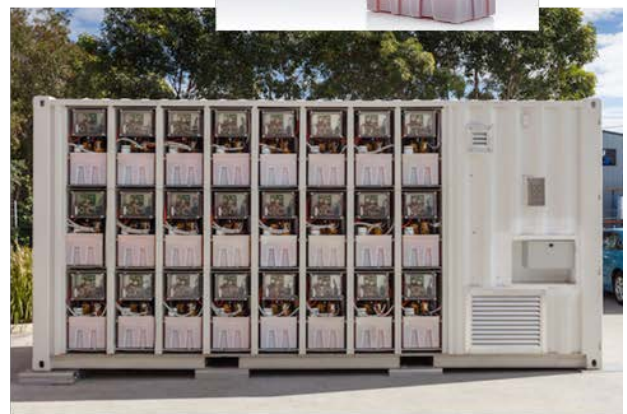
Redflow Zn-Br 2 system (300 kW / 660 kWh; container de 20 feet, 25 t) http://www.impress.com.au/newsroom/redflow/1933-redflow-powers-up-for-battery-battleground.html
