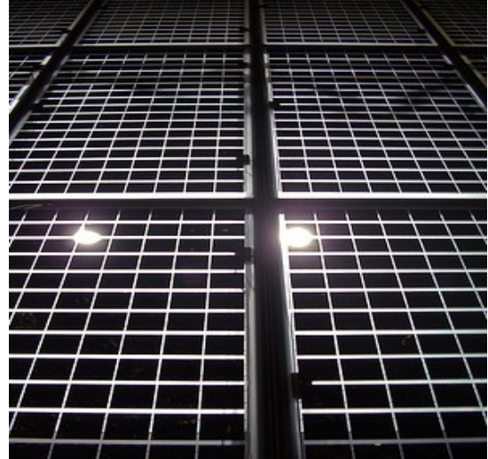
Figure 6.2 Daylight entering via the openings between the cells
