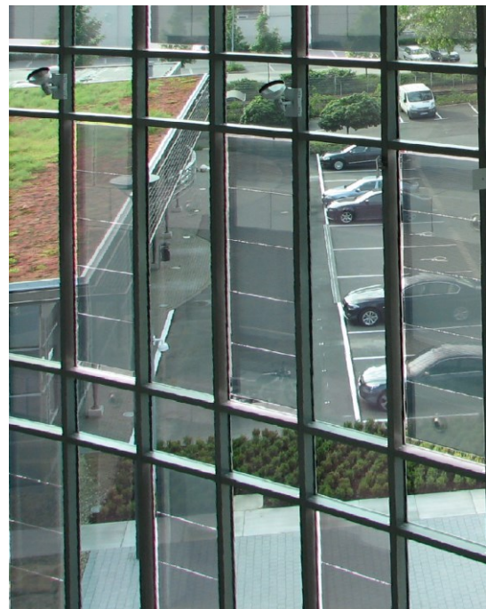
Figure 7.14 Almost invisible solar modules. □ Schott Solar ASI Thru modules.
