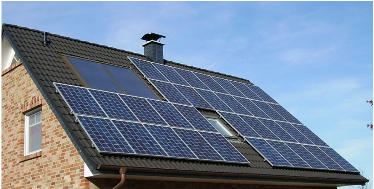
Figure 7.3 Typical BAPV solution of the type 'asymmetrical/area'
