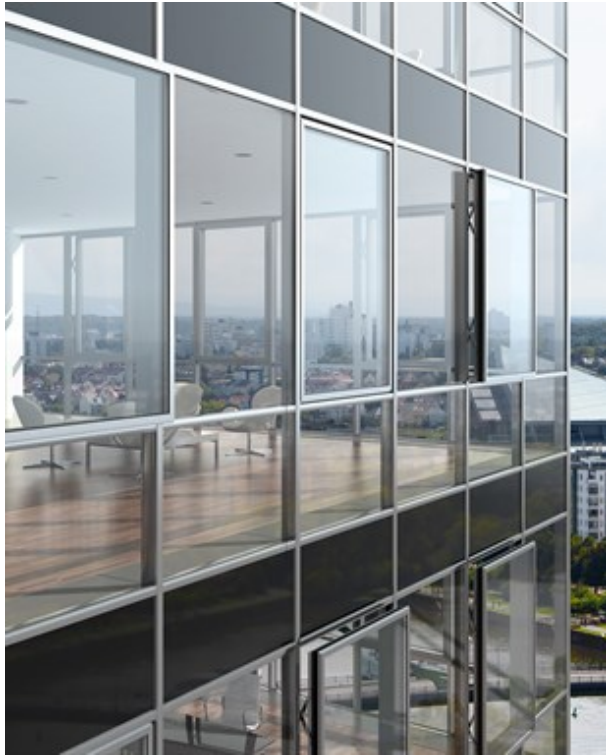
Figure 6.12 Facade system: frame. Non-structural panels in frames
