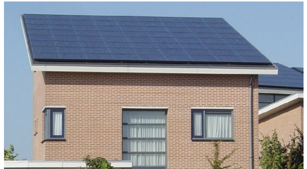
Figure 7.9 Almost invisible mounting with Alutec profiles. Langedijk-1 Meyersloot. □ Design BEAR-iD, Tjerk Reijenga.
