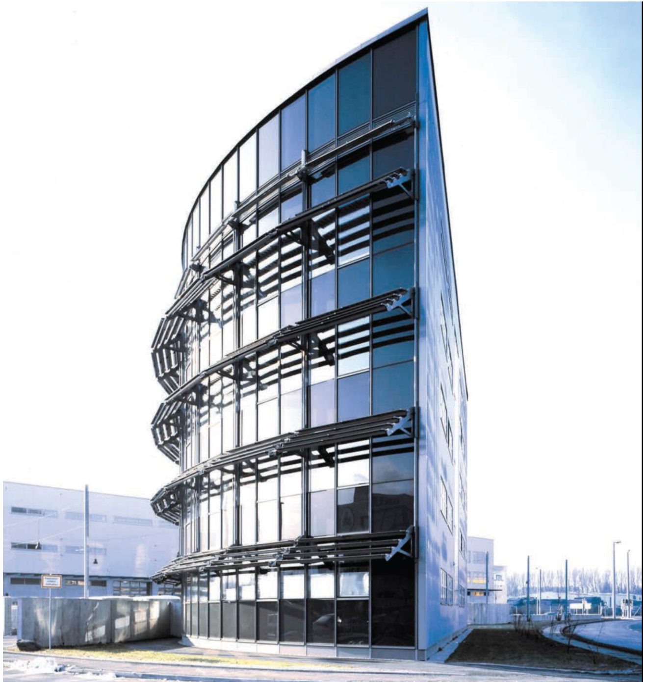
Figure 3.7 SBL Offices Linz Austria. Sunshading: Colt
