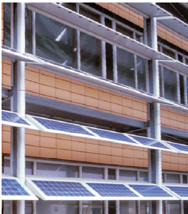
Figure 6.10 Horizontale shading with solar modules. ECN building 31, Petten (NL). Design: BEAR-iD, Tjerk Reijenga
