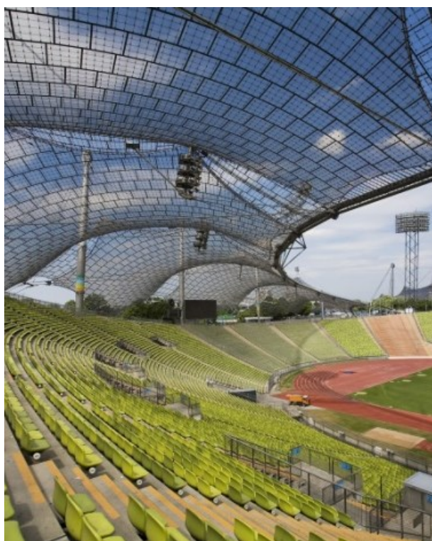
Figure 6.16 Roof system: Tensegrity. Olympiapark, München; design: Frei Otto
