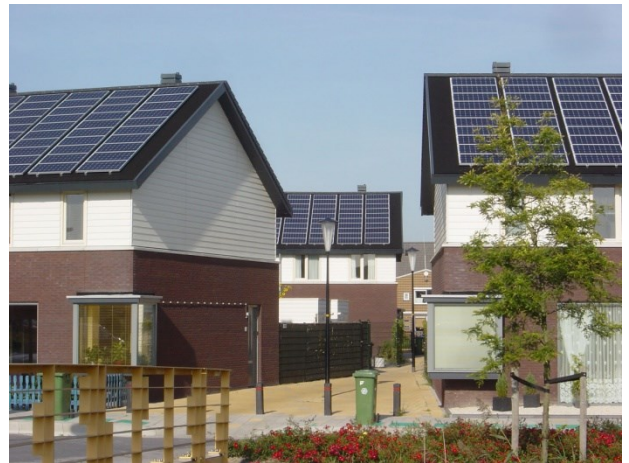
Figure 9.6 The layout of the PV-modules on this roof is not designed. The edges and rim of the roof are clearly visible. The result is not very aesthetical. City of the Sun, Heerhugowaard
