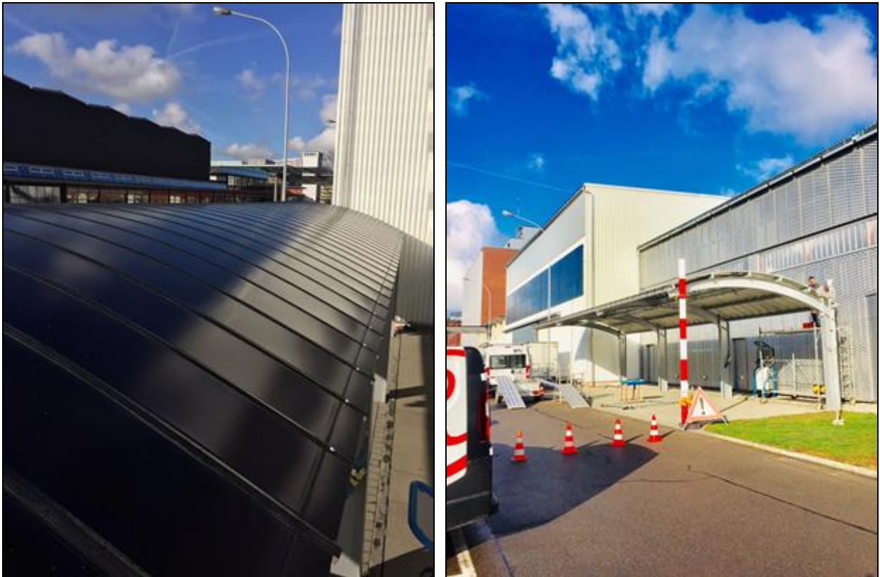
Figure 5.4: Carport modules installed on demo-site EMPA
