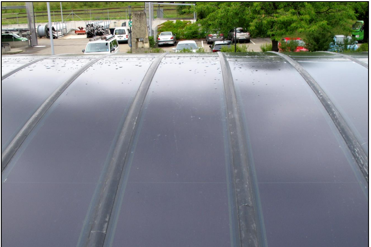
Figure 5.3: Carport modules installed on demo-site EKZ Seuzach
