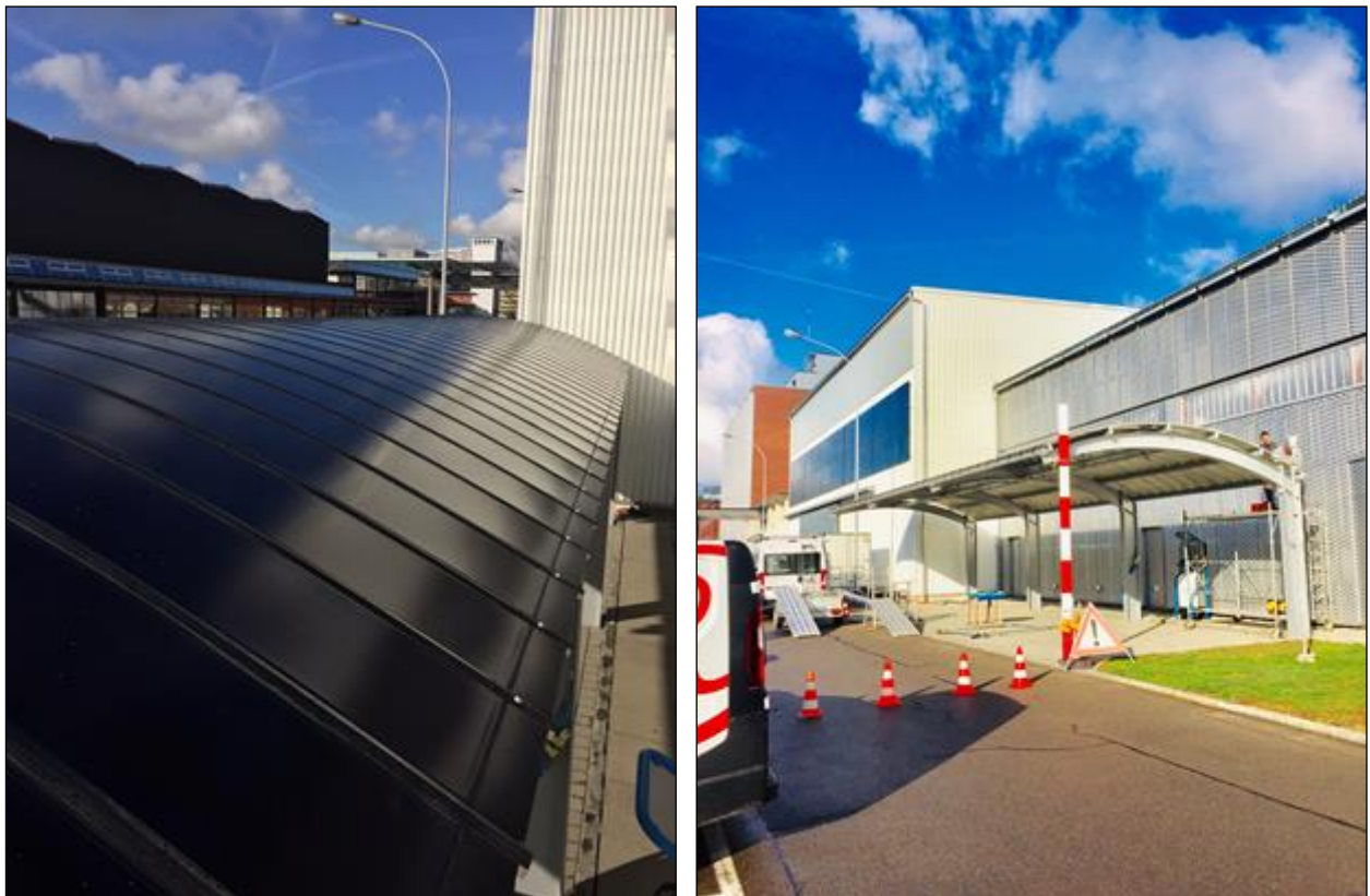
Figure 4.4: Carport modules installed on demo-site EMPA
