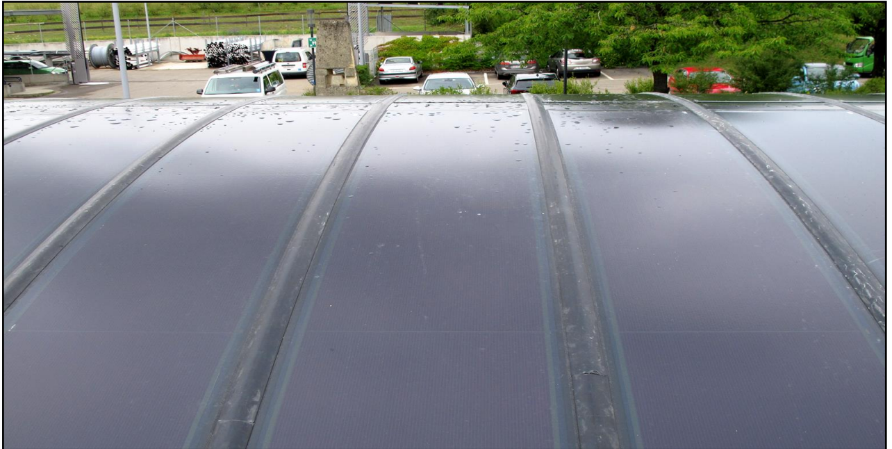
Figure 4.3: Carport modules installed on demo-site EKZ Seuzach
