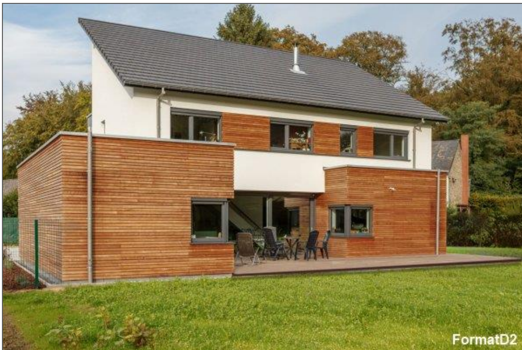
Figure 3.1: Demo 1. FORMAT D2 residential and professional building in Belgium
