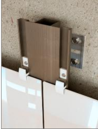
Figure 3.46: “SB fijaciones” clip system and real application for a glass-panels facade
