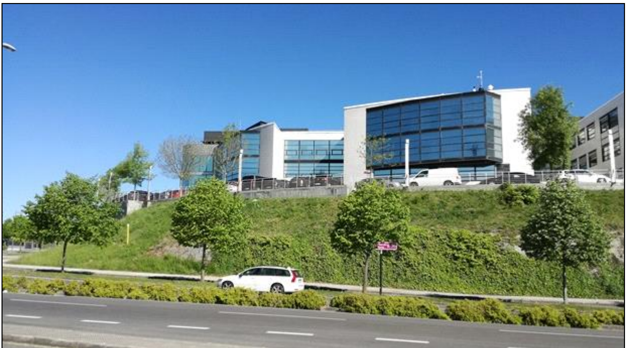
Figure 3.47: TECNALIA offices and labs in San Sebastian
