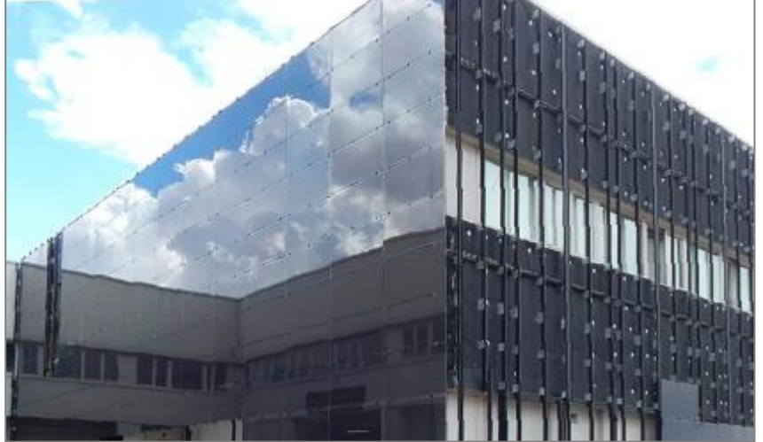
Figure 3.46: “SB fijaciones” clip system and real application for a glass-panels facade
