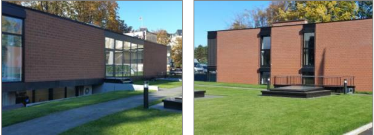
Figure 3.10: East and West façades of the Pavilions 1 and 2, respectively
