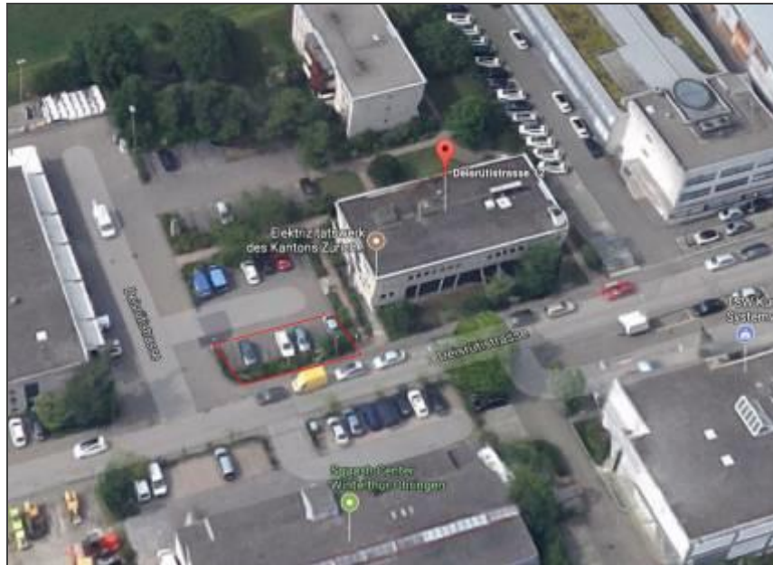
Figure 3.18: Location of one of the demonstrative PV carports in EKZ facilities, Switzerland
