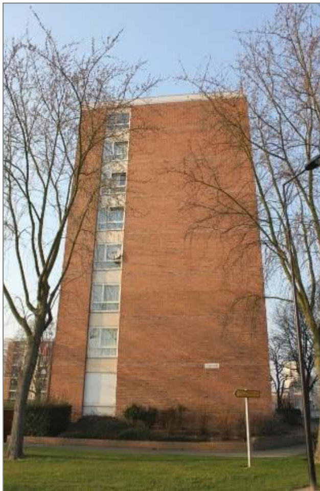
Figure 3.40: Demo 5. Residential 8-storey building, provided by VILOGIA
