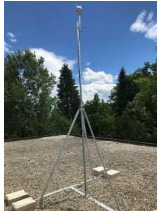
Figure 3.7 Weather station and pyranometer installed on the roof of Pavilion 2
