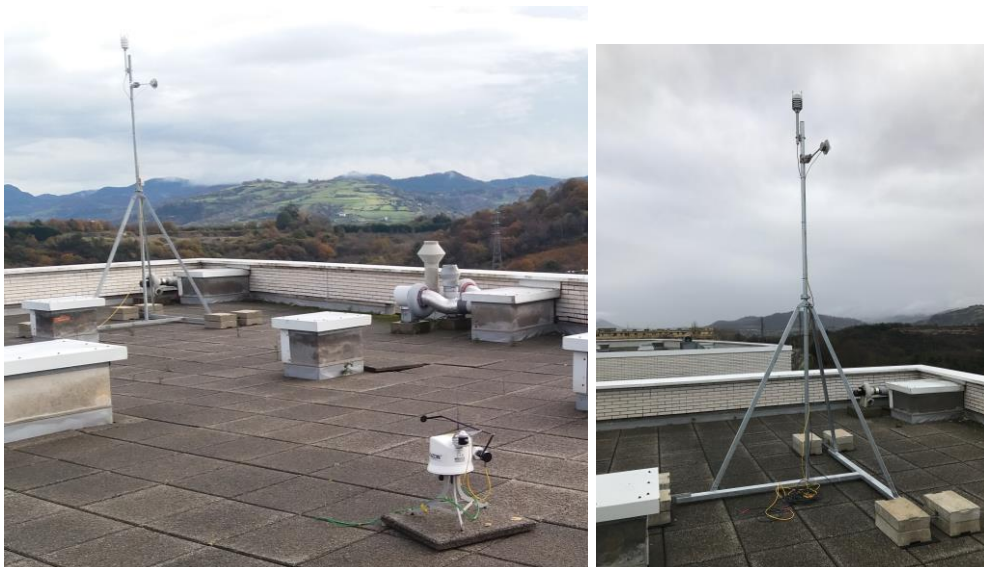
Figure 3.23 Weather station and solar tracker installed on the roof of TECNALIA building
