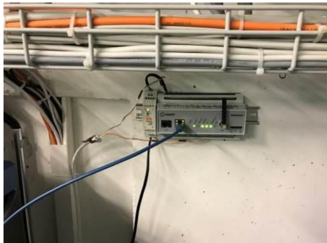
Figure 3.8 Gateway WebdynSun installed in server room on the ground floor of Pavilion 2 (picture on the left) and Gateway WebdynSun installed in ventilation room on the ground floor close to Pavilion 1
