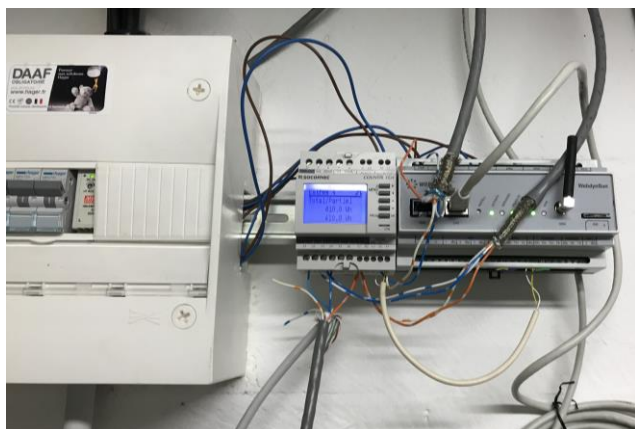
Figure 3.19 Gateway associated with the weather station
