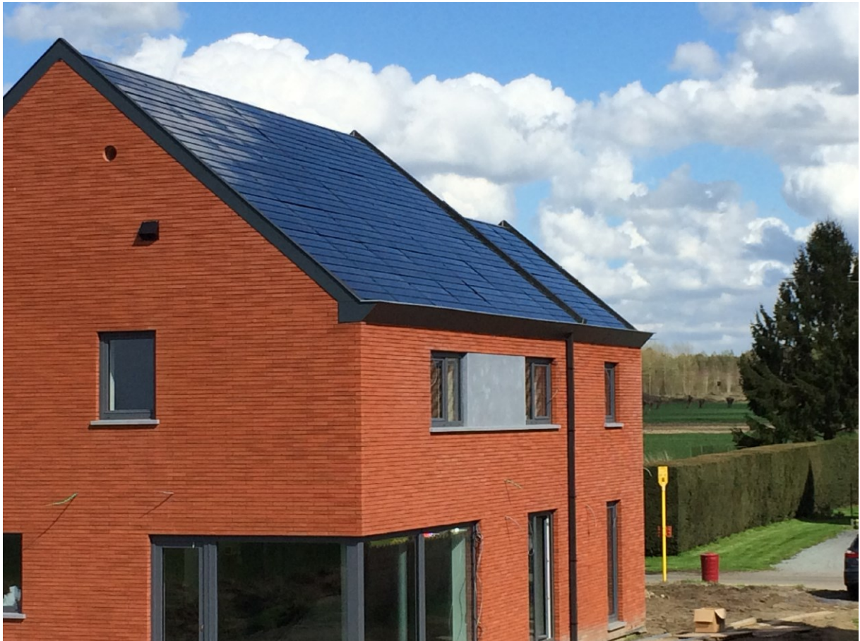
Figure 26: Single family house in Belgium Flanders with 46 m 2 BIPV roof [design Format D2, Dominique Deramaix, roof elements from BFIRST FP7 project, Grant Agreement 296016].
