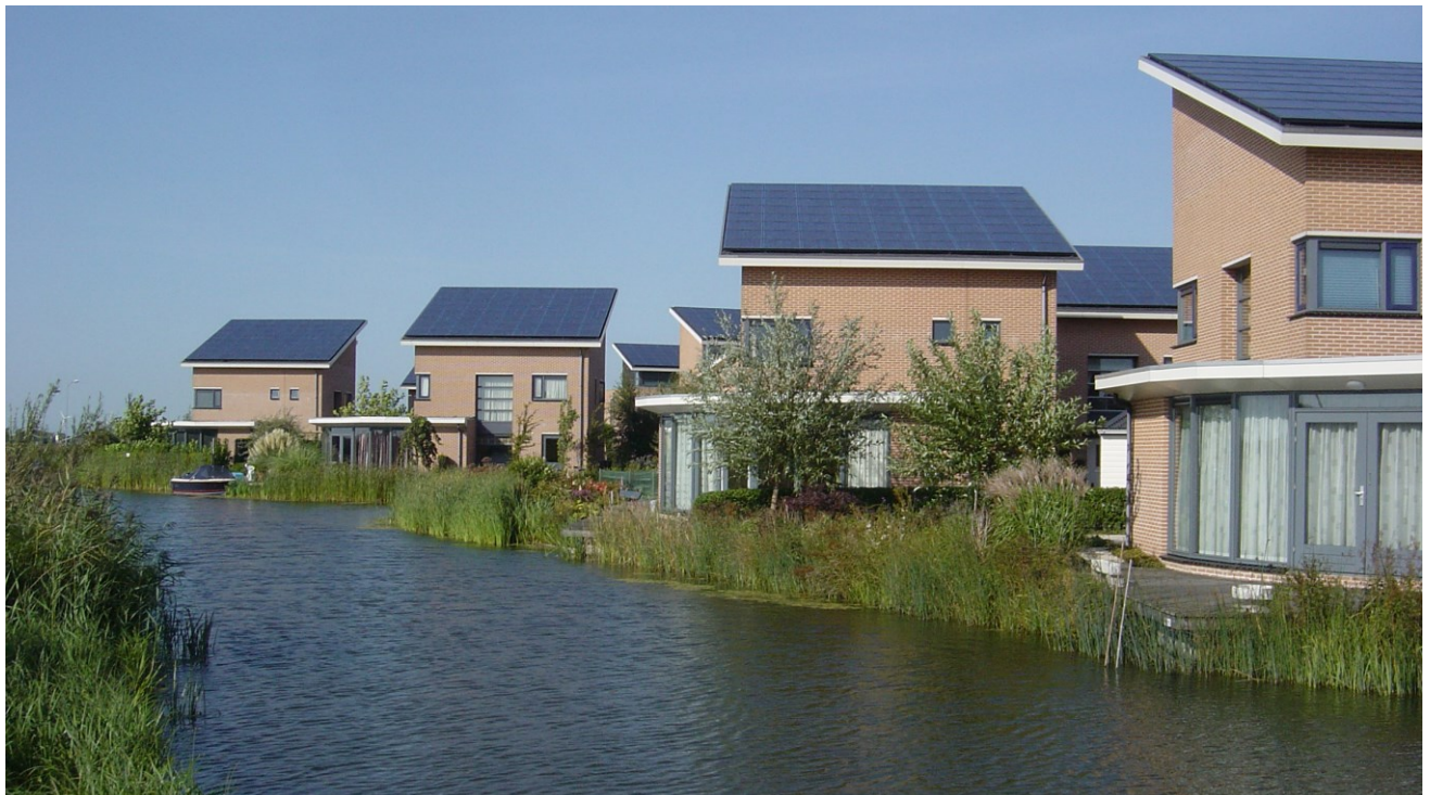
Figure 25: Single family houses with large (60 m 2 ) PV roofs [design BEAR-iD, Tjerk Reijenga].
