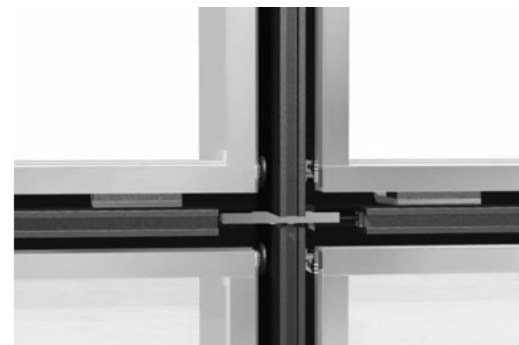
4. Place the glass over the structure
