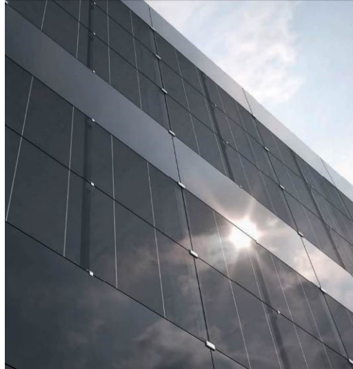
Figure 2.4 Integration example of S-Vitech FP4001PV ventilated façade system. Source: Vitech/Silva&Ventura
