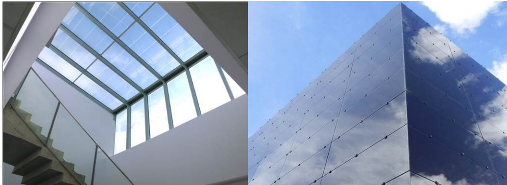
Figure 2.1 BIPV skylight and curtain wall (left) and BIPV ventilated façade (right). Source: ONYX
