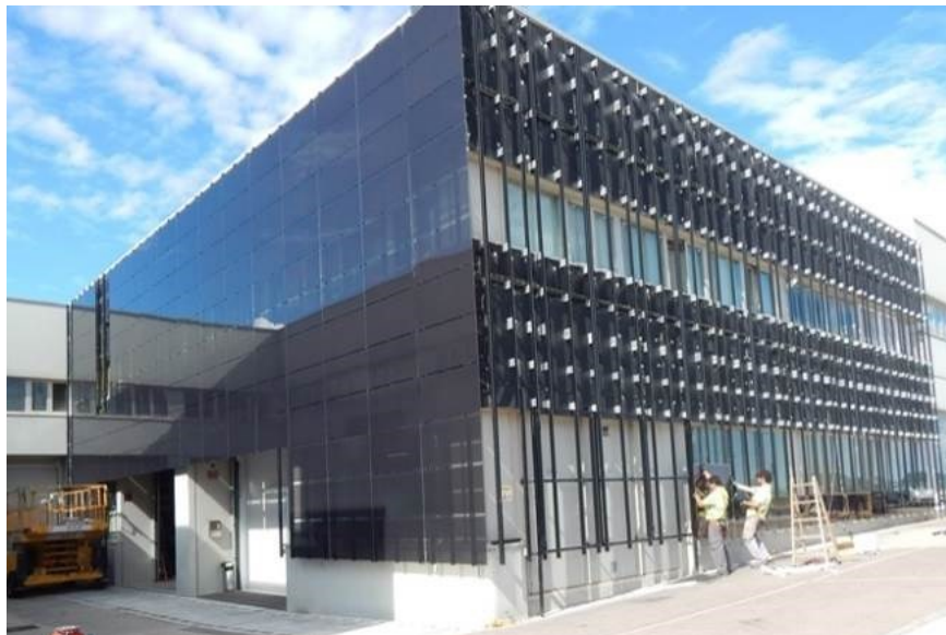
Figure 2.8 PV ventilated façade project in ONYXS’s HQs (Ávila) using SB Fijaciones system. Source: SB Fijaciones/ONYX)
