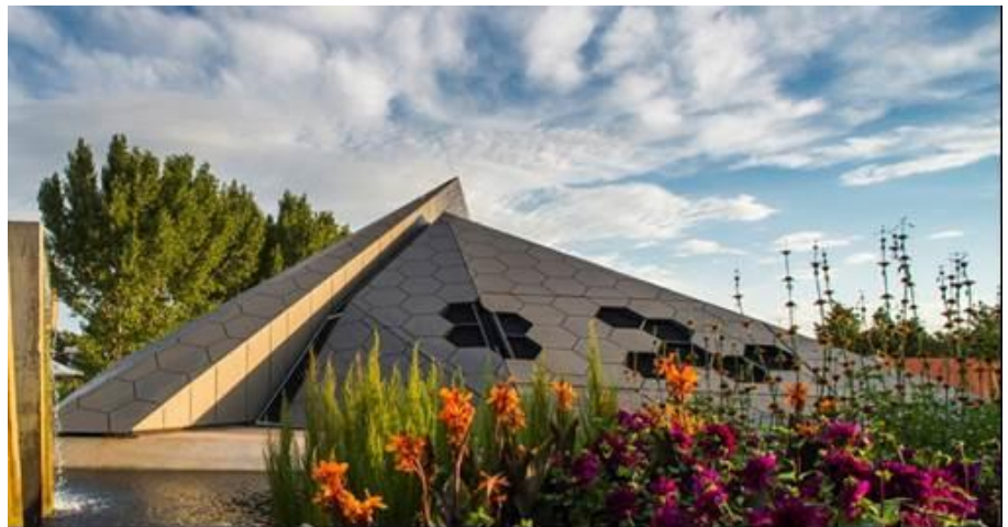
Figure 2.3: Vented cladding on Botanic garden of Denver
