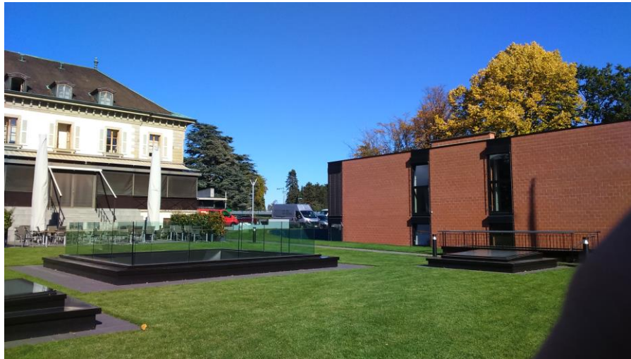
Figure 5.3: One of the buildings in EHG site involved in the demonstration (right side of the photo)
