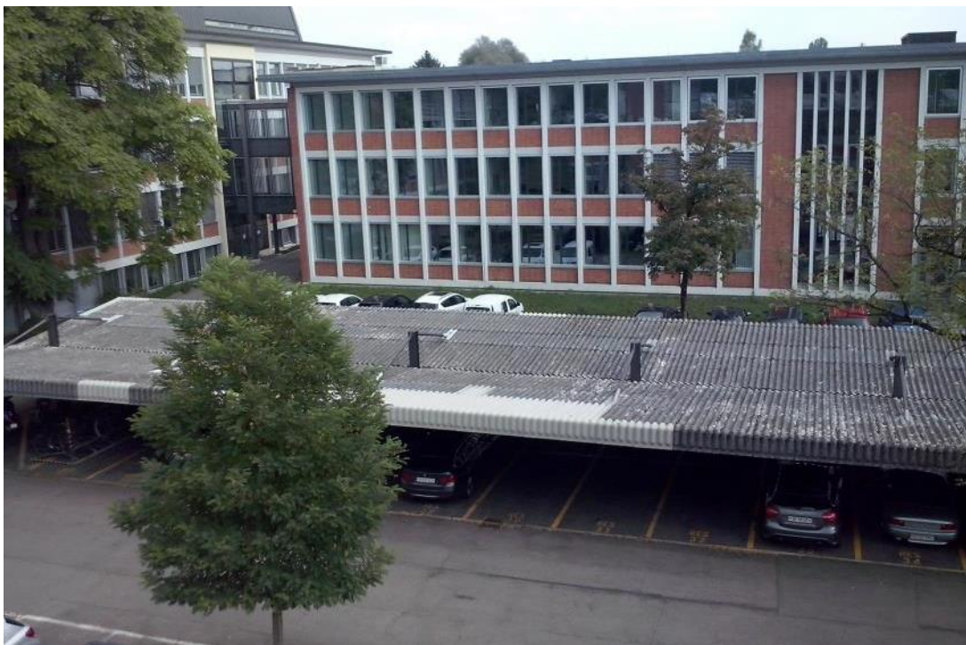
Figure 4.10 Overview of the carport located in the EMPA facilities
