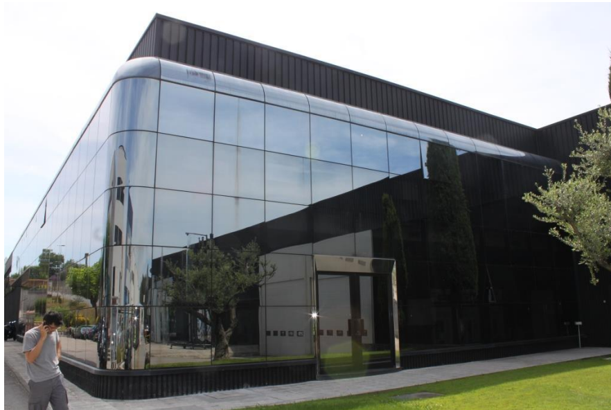
Figure 3.4 Industrial and offices building complex in Spain, provided by CRICURSA.
