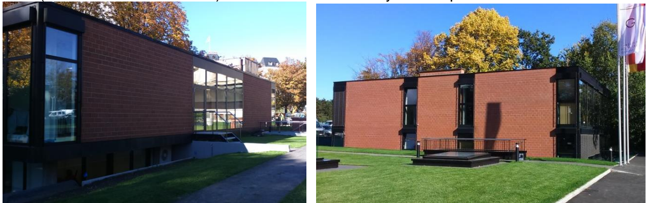
Figure 4.6 West and East façades of the pavilion 1 and 2, respectively
