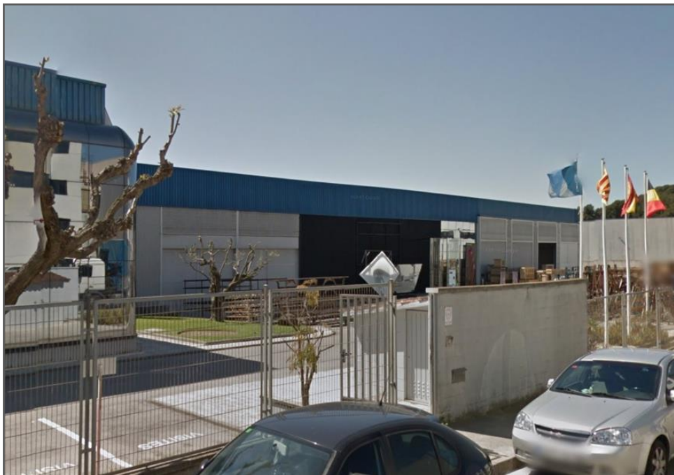
Figure 2.7 DEMO#4 – CRICURSA, Industrial and office building complex in Spain
