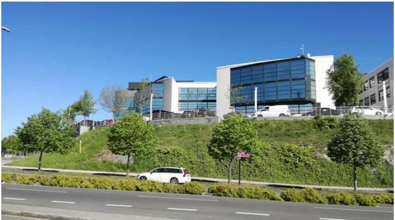
Figure 2.11: DEMO#6 – TECNALIA offices and labs in San Sebastian
