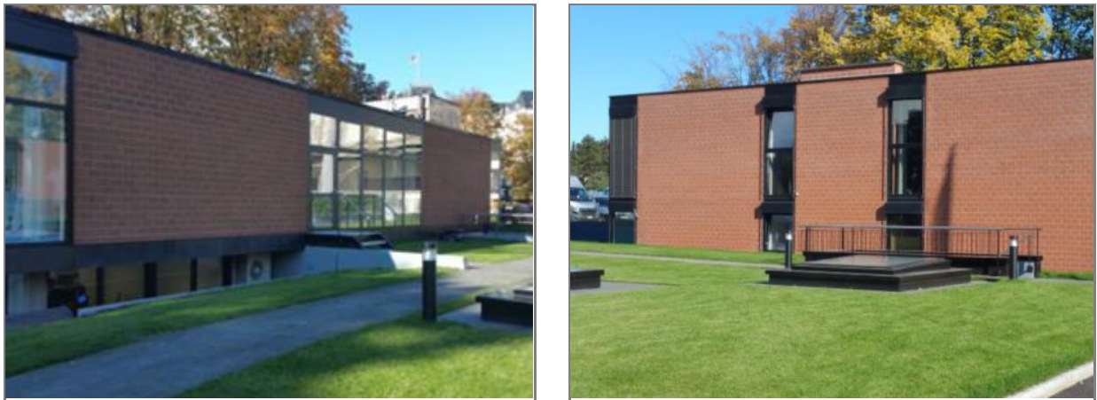
Figure 2.4: DEMO#2 –EHG East and West façades of the Pavilions 1 and 2, respectively
