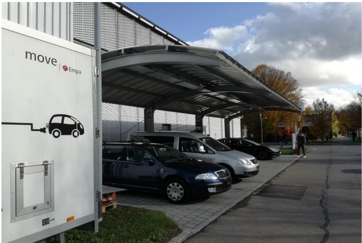
Figure 5.1: Final results of Demo-system 3, EMPA's Carport in Switzerland
