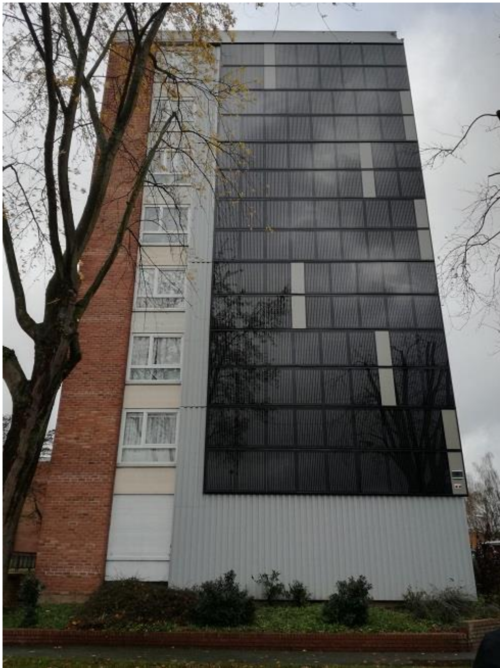
Figure 7.1: Final results of Demo-system 5, Apartments Building in France
