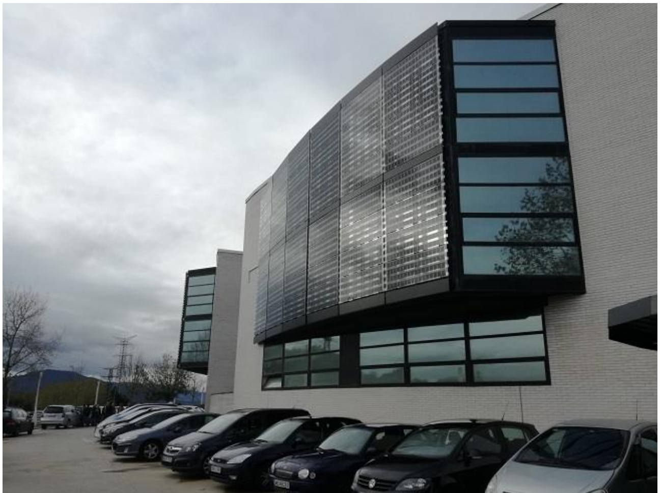
Figure 8.1: Final results of Demo-system 6, Office Building in Spain
