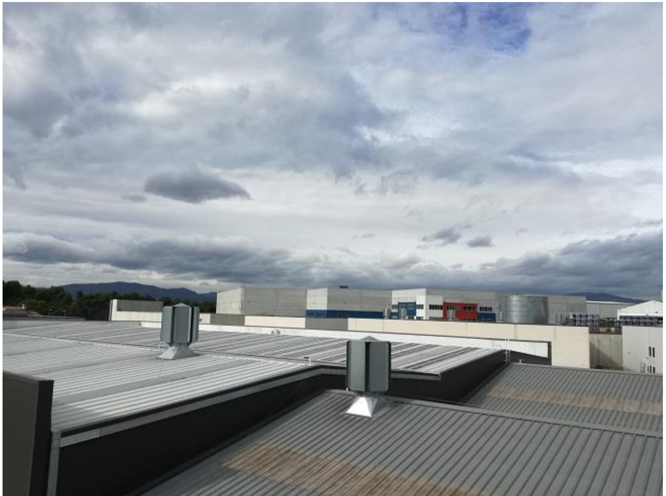
Figure 6.1: Final results of Demo-system 4, Industrial Building in Spain
