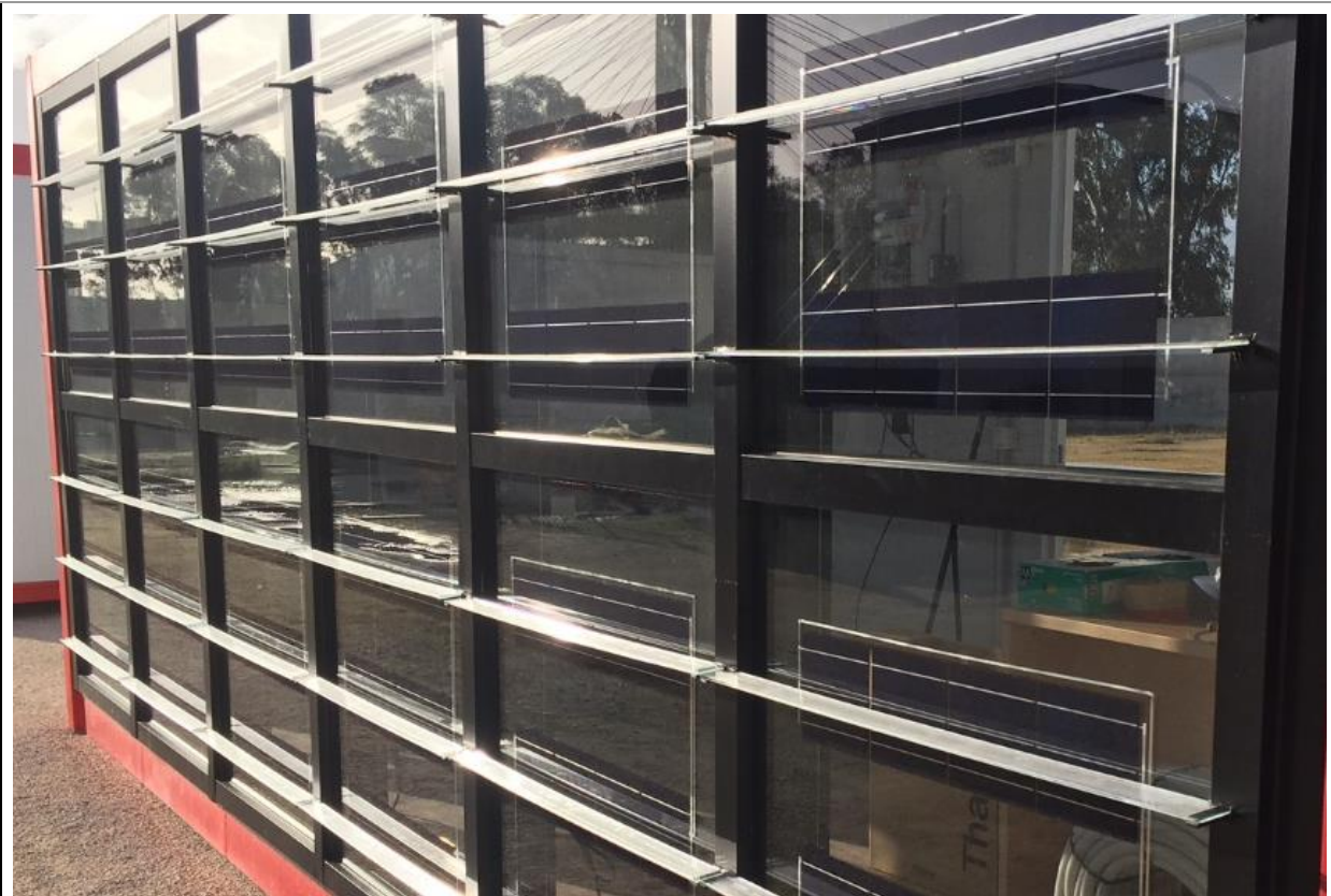
Façade integration detail with lenses
