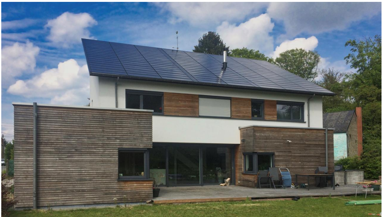
The house after the roof renovation with BIPV shingles.
