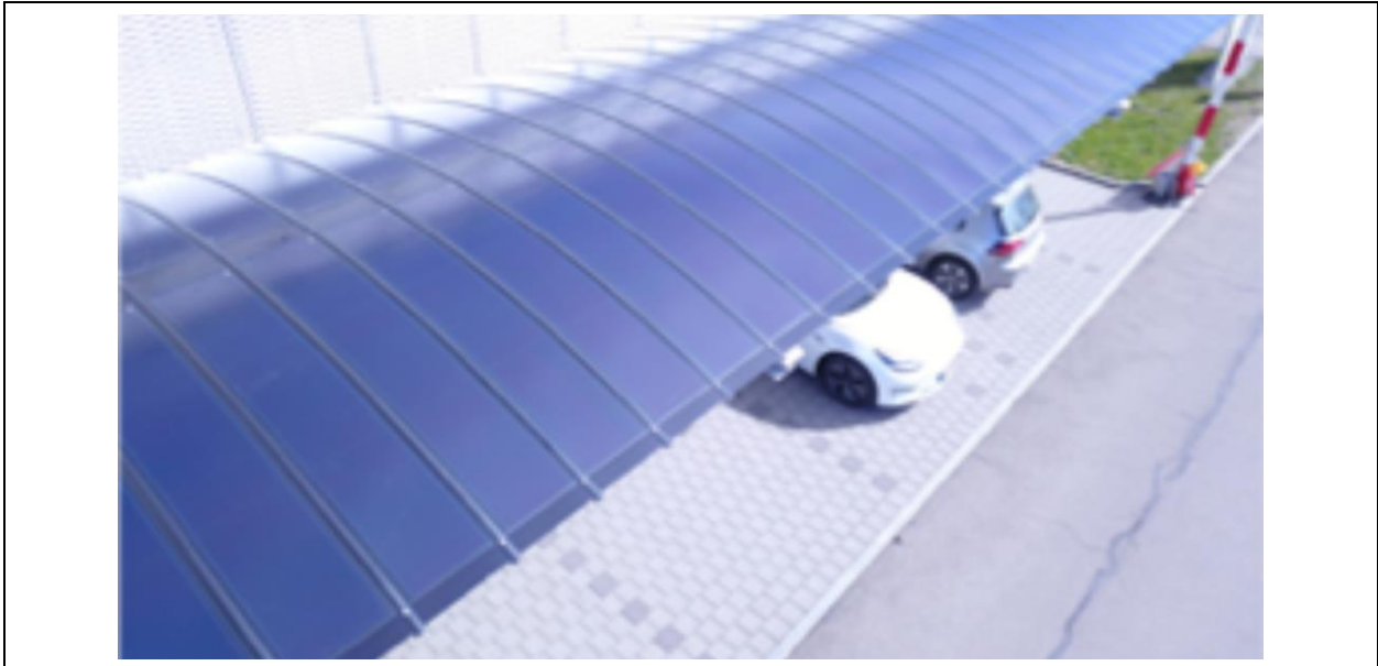
Carport at EMPA Zürich after construction.
