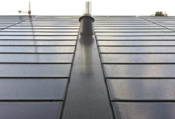
PV roof tiles on demo site in Belgium
